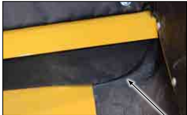
Fig 104 - New side flashing
