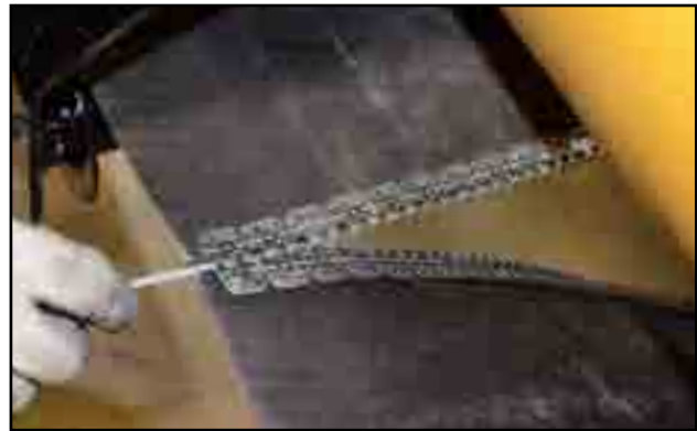
Fig 97 - Thread lacing cable
