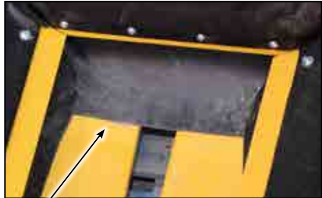
Fig 103 - New tail flashing
